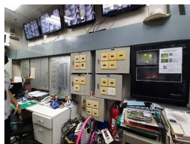
Graphic Annunciator Fire Alarm System
